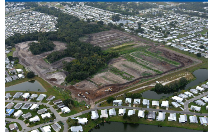
Colony Cove – Ellenton, FL Completed Expansion Sites
