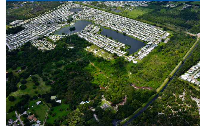
Buccaneer Estates – North Fort Myers, FL Expansion in Progress
