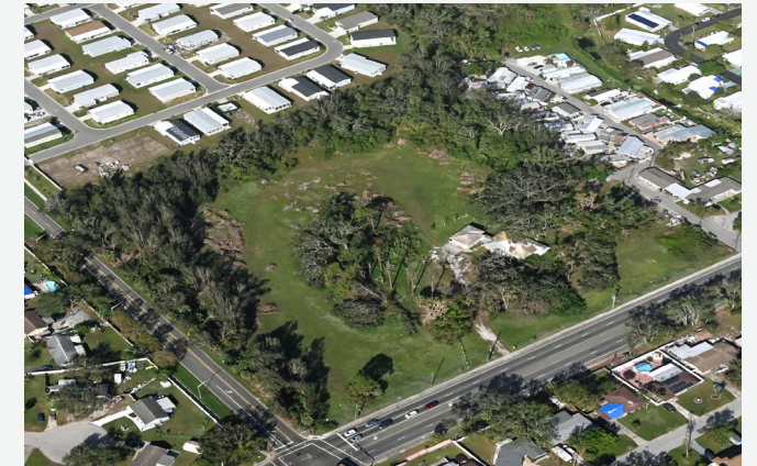
Winds of St. Armands South – Sarasota, FL Expansion in Progress
